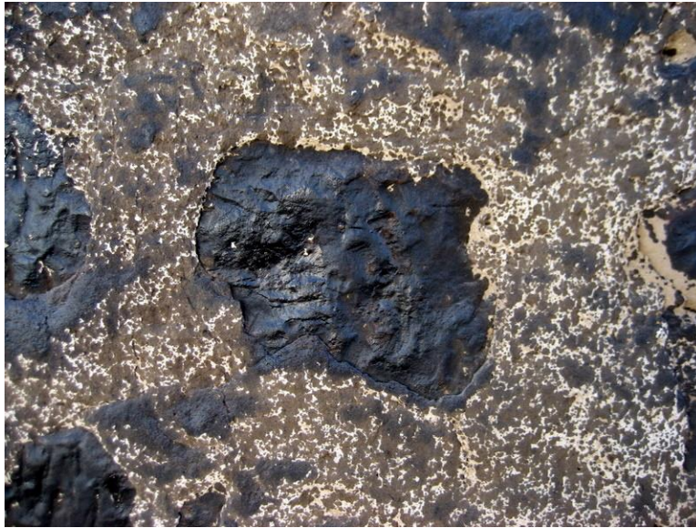
figure 1. typical wall condition following asphaltic application
