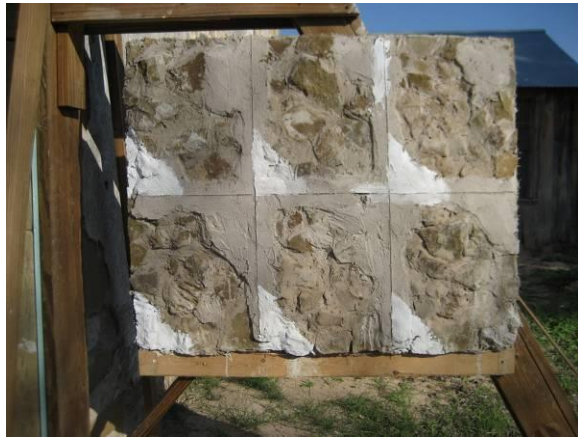
figure 5. test panel before MC-30 application
