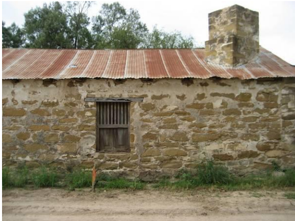
figure 2. N facade, Kitchen #2 July 2009
