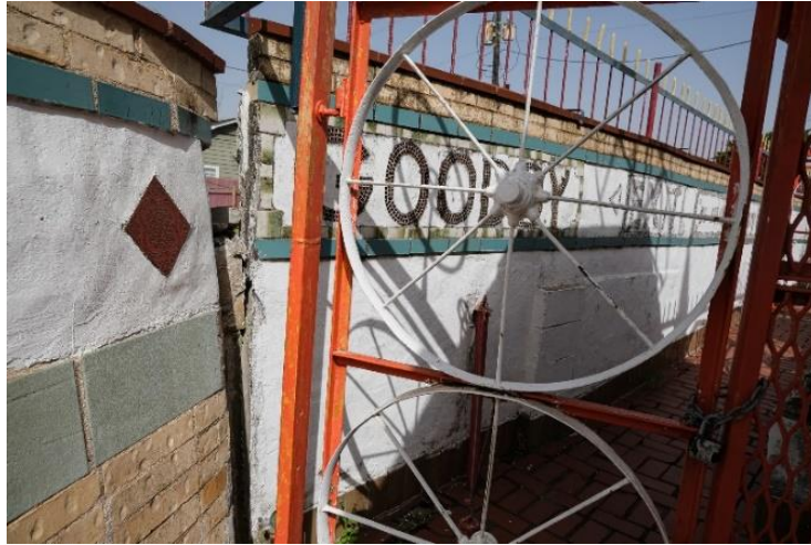
Figure 13. Additional break in an unreinforced single-wythe solid masonry wall.
