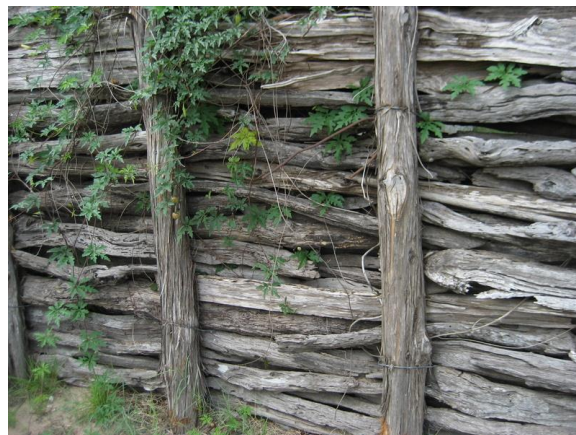
figure 27. cedar posts with mesquite infill, typical
