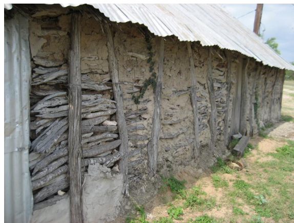
figure 12. north façade of Bunkhouse, repair at left post
