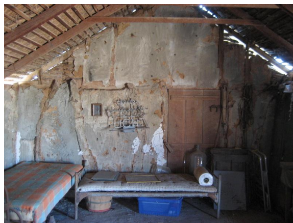
figure 16. Bunkhouse interior looking east
