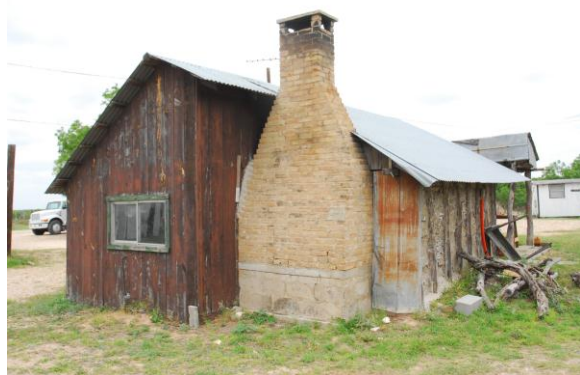
figure 20. Kitchen jacal, west façade with chimney
