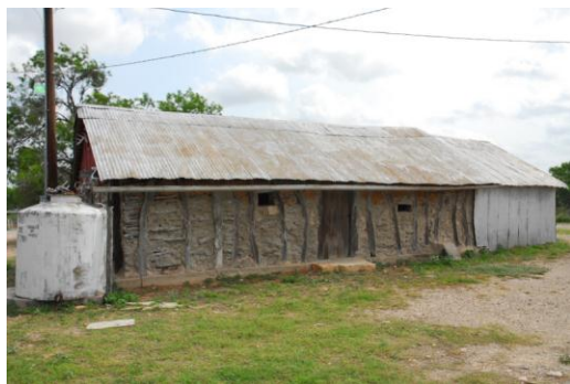
figure 7. Old Bunkhouse jaca, south facade
