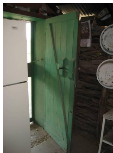
figure 22. plank door with wood latch
