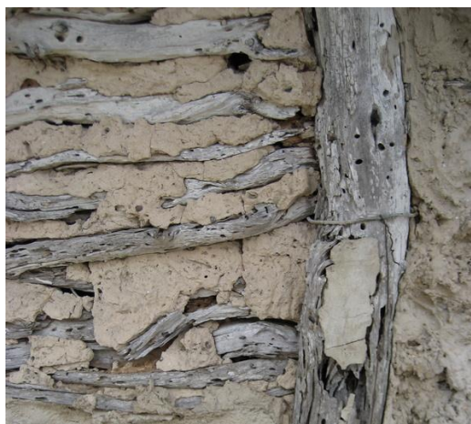
figure 8. typical Bunkhouse exterior wall construction
