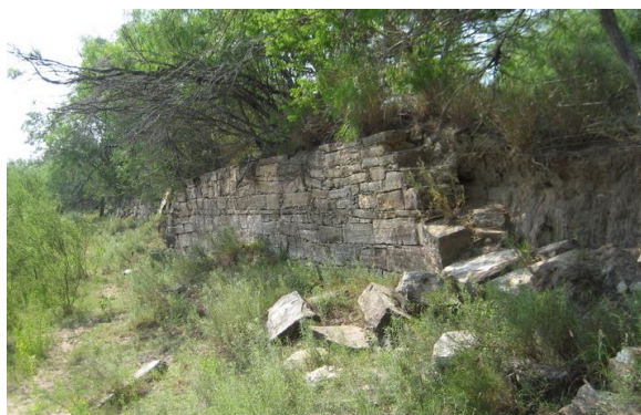
figure 5. a tall section of the stone dam
