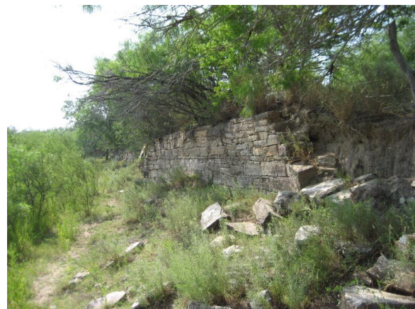
figure 25. tallest section of the dam, about 7'6"
