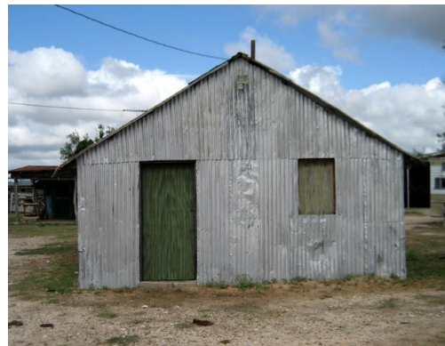
figure 10. east façade Bunkhouse addition
