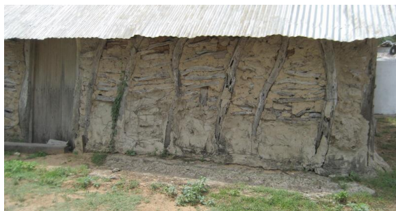
figure 29. cement plaster at wall base near northwest corner
