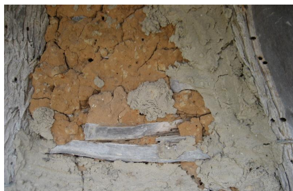
figure 14. early reddish and tan plasters below cement
