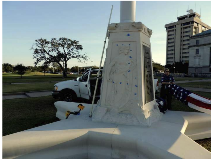
Monument during determination of rebar locations.
